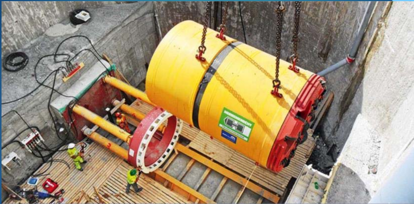
MACHINE INTRODUCED TO JACKING PIT
