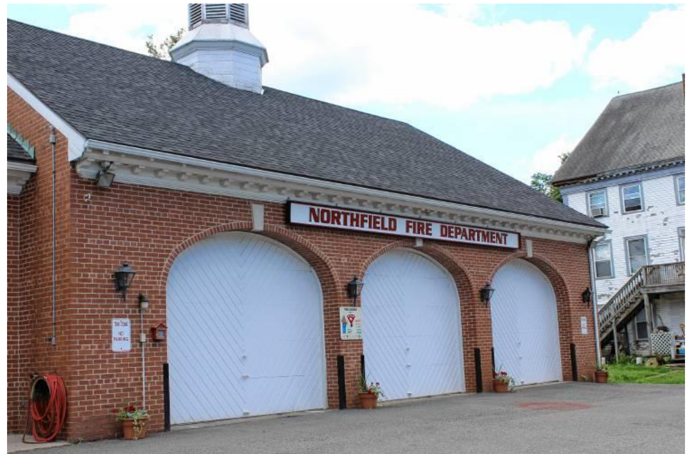
The existing fire department building
