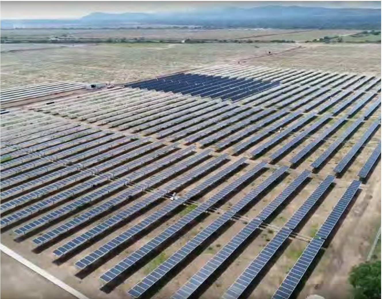
MEXICO Santiago & Hermosillo, 170+100MW HEC V1500 + MV SKID
