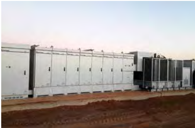
JORDAN Al Mafrq, 61MW HEC V1500 + MV SKID JORDAN'S 1 ST 1500V INVERTER
