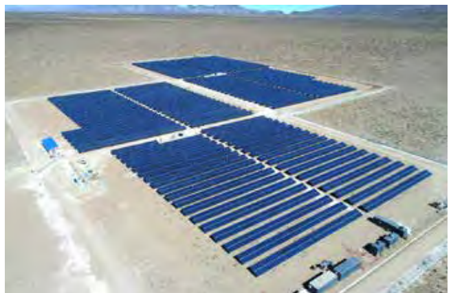
BOLIVIA Uyuni & Yunchara, 60+5MW HEC V1500 + MV SKID BOLIVIA 1 ST 1500V INVERTER
